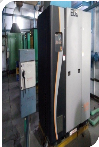
VFD's for Compressors
