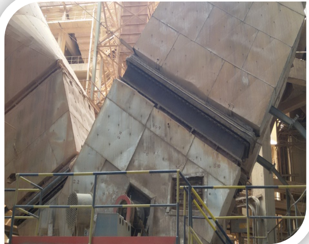
Preheater Fan Damper removal in Line-2
