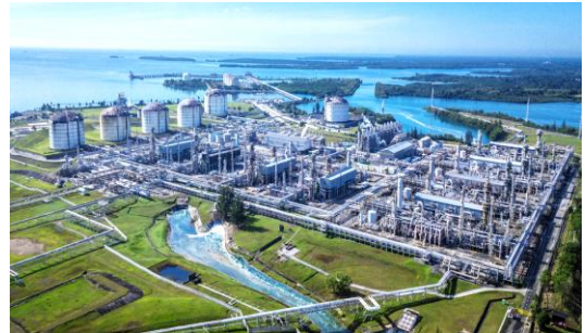
Figure 1 PT Badak NGL Plant Site – Bontang,
